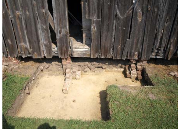
Figure 4: View of T.U. 13 (left) and 14 showing the remains of the chimney foundation.
